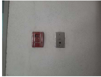
Fire Alarm Manual Station
