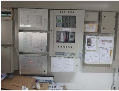
Graphic Annunciator Fire Alarm System
